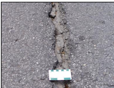
Figure 2.c Severe Longitudinal Cracking
