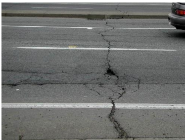
Figure 3c Severe Transverse Cracking
