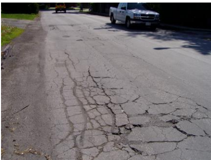
Figure 4c Severe Alligator Cracking
