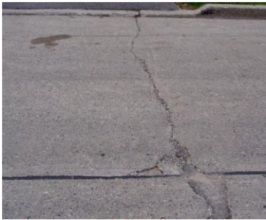
Figure 3a Slight Transverse Cracking
