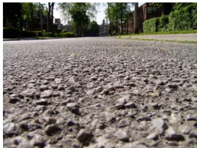
Figure 1c Severe Raveling
