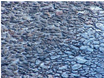
Figure 1b Moderate Raveling
