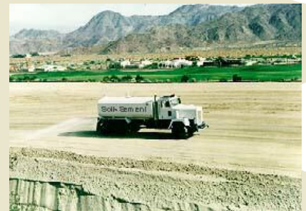
Soil-Sement® applied to a construction site ...
